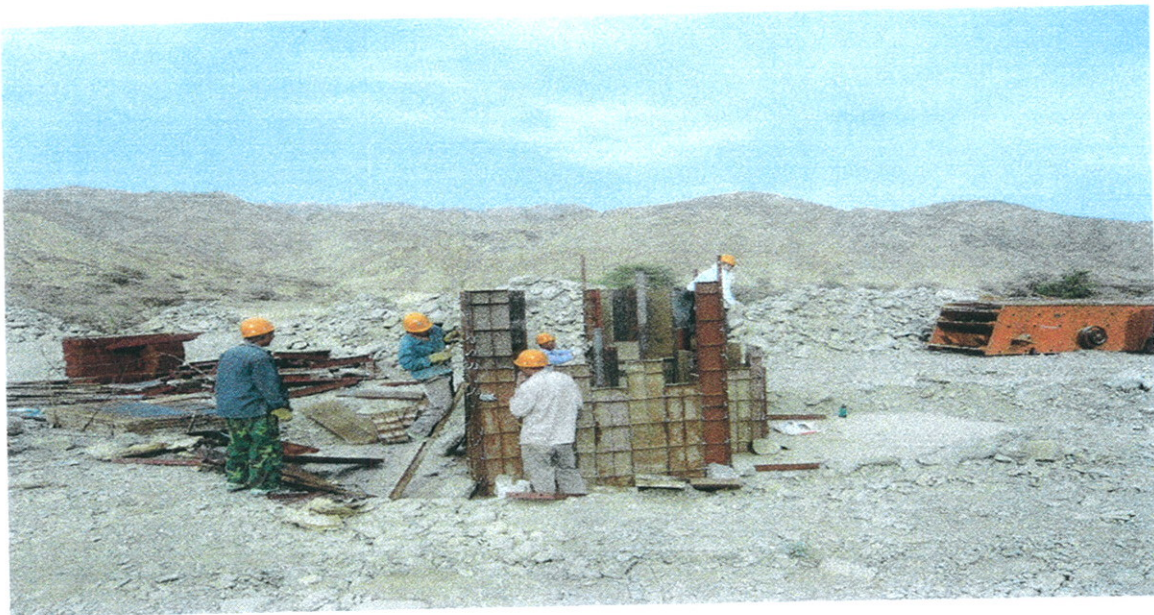
Temporary Crusher Plant
