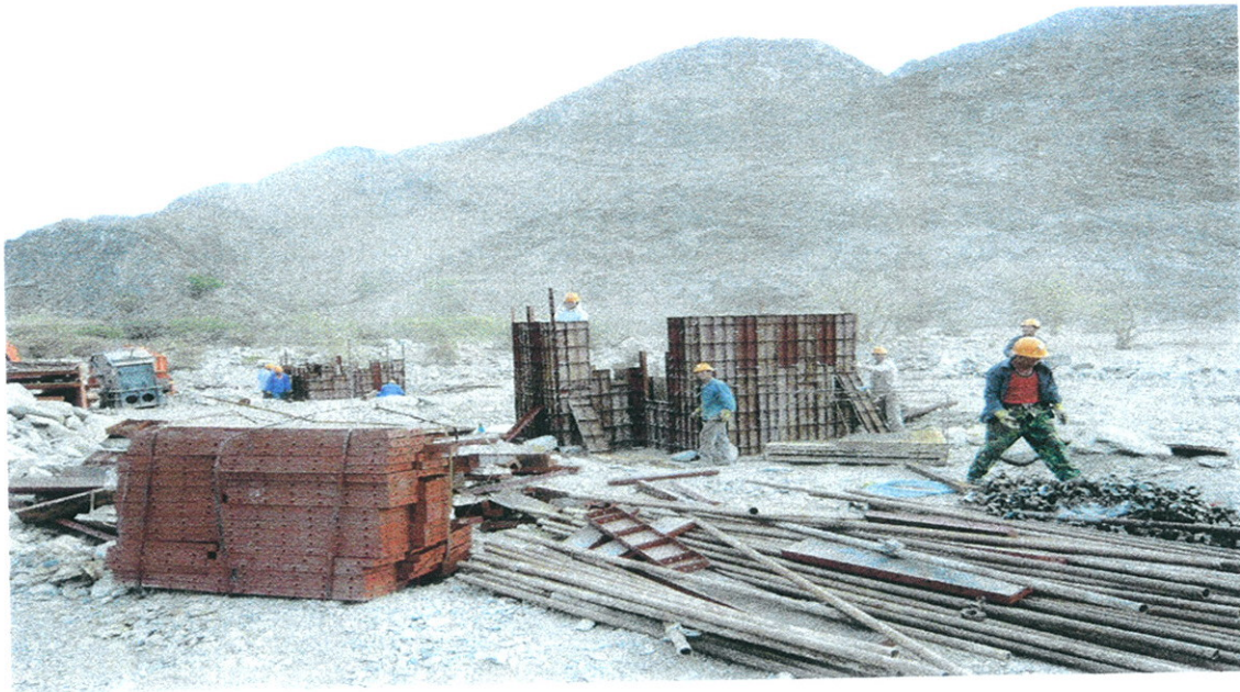
Temporary Crusher Plant
